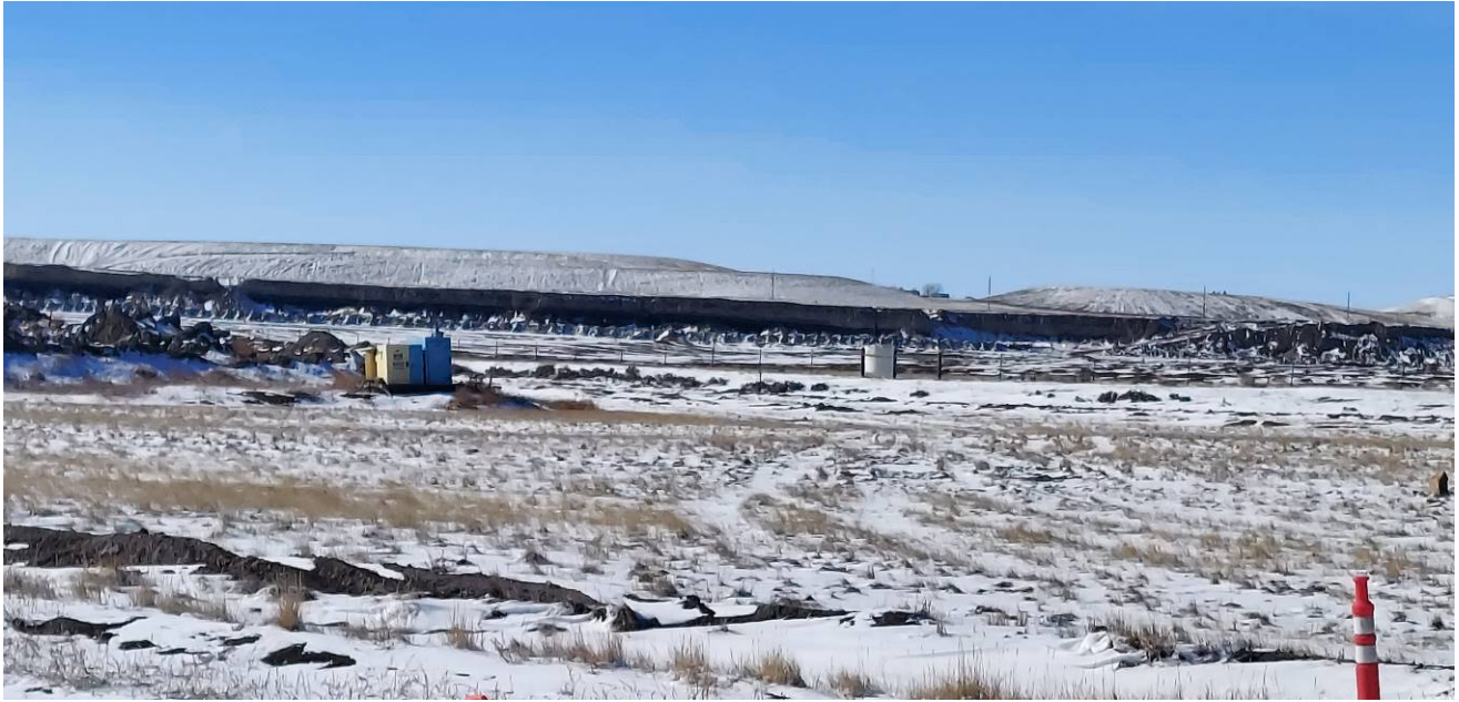
Photo #3 – Looking west at approximate mid-point of new alignment
