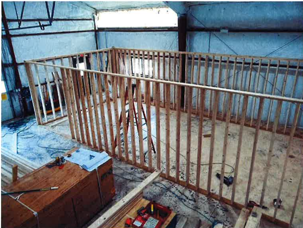
Figures 1 and 2. Rockpile Museum Annex and construction of a new climate-controlled collections storage room in 2020.
