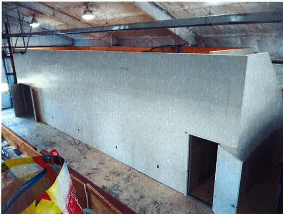
Figures 3 and 4. Interior and exterior of the completed storage room constructed in 2020.
